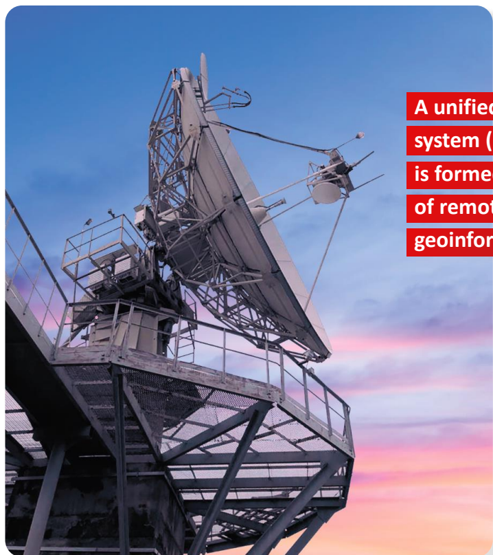
Ground relay reception complex (GRRC)
